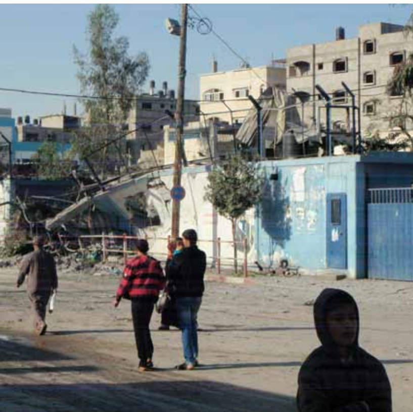
◀ Debris of the building of the Council of Ministers in Gaza City
