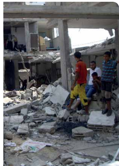
Houses that were destroyed in Deir al-Balah in the central Gaza Strip as a result of an explosion that occurred on 5 August 2010
