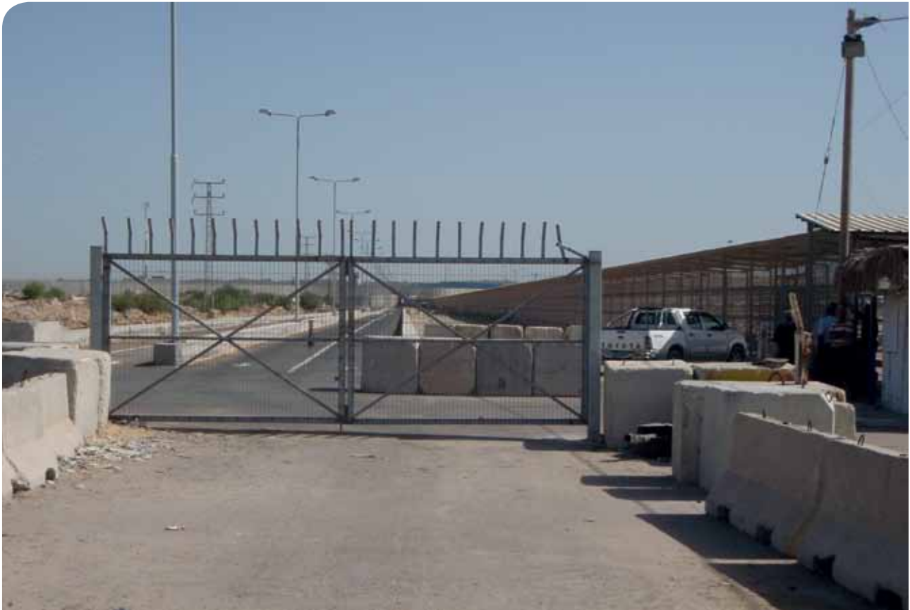
Beit Hanoun (Erez) Crossing in the far north of the Gaza Strip
