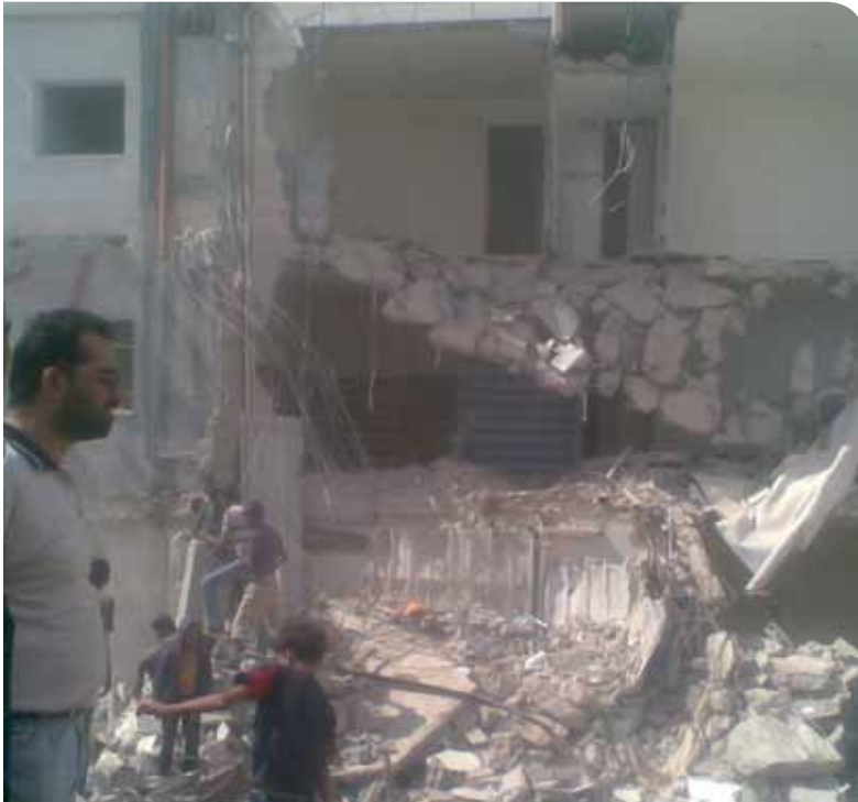
House demolitions in the West Bank.
