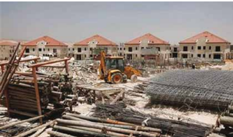
Construction works in an Israeli settlement in the West Bank.
