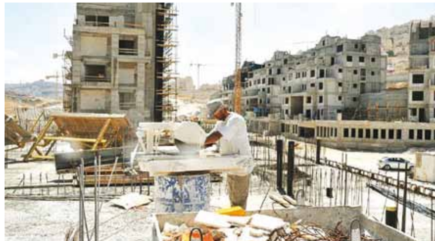
Construction works in "Pisgat Ze'ev" settlement, in East Jerusalem.
