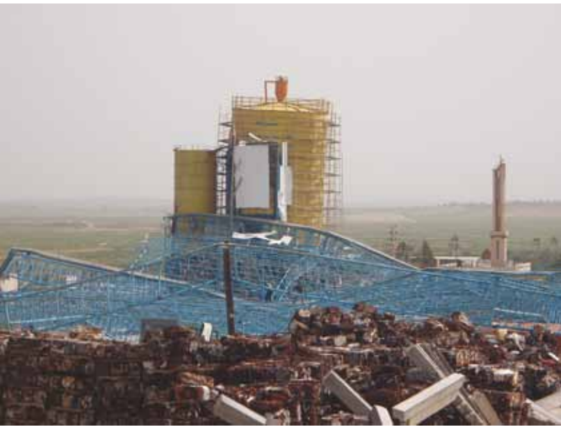
Abu Jubba Concrete Factory, which was destroyed by IOF in the east of Gaza City.
