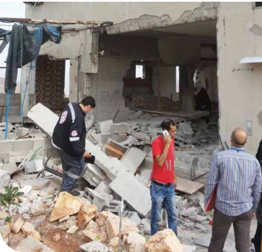
Israeli forces demolish a house in Nablus
