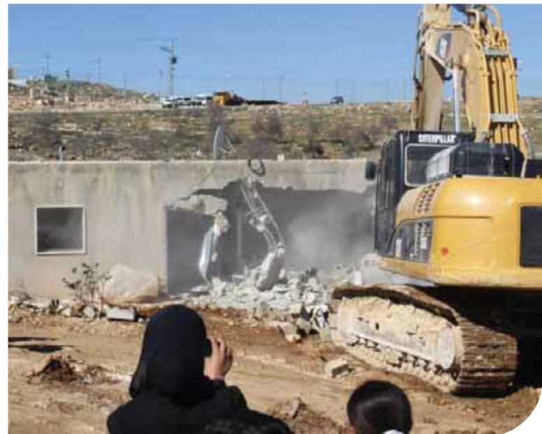
Israeli forces demolish a house in Yatta on 22 January
